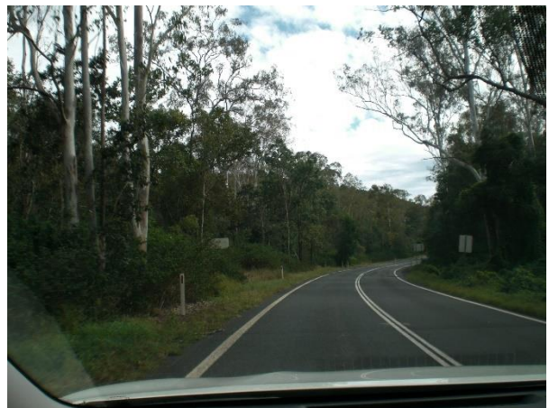
Narrow with roadside hazards (south of Blackbutt Range)
