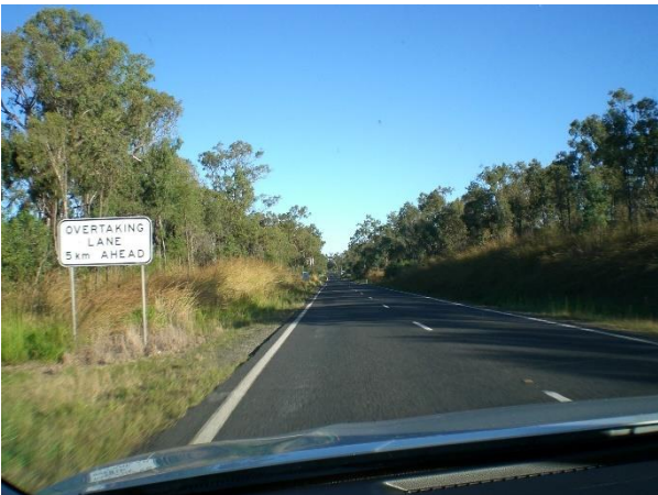
Narrow section near Kolonga for ~15km
