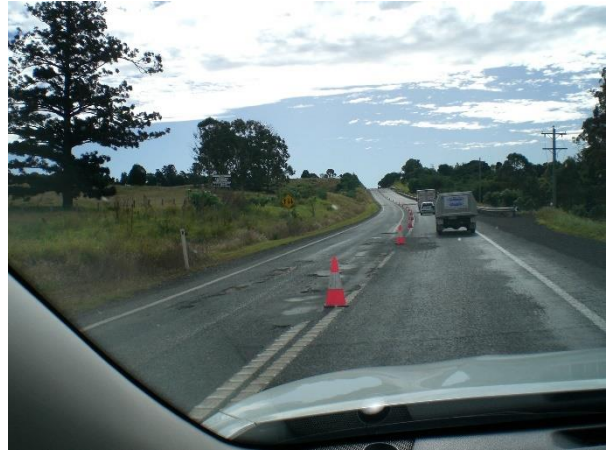
Pavement failures
