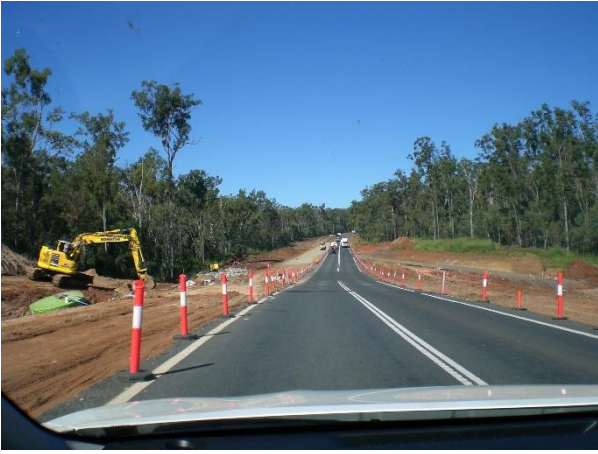
Roadworks upgrade project
