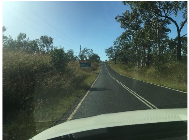
Narrow lane and narrow shoulders
