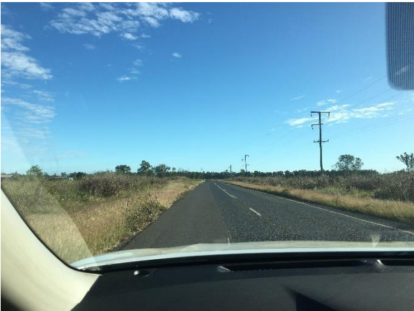
Narrow lane and no shoulders
