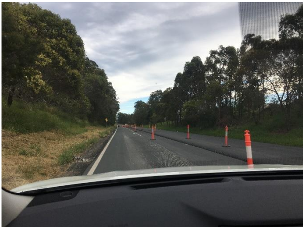
Roadworks at Wamuran
