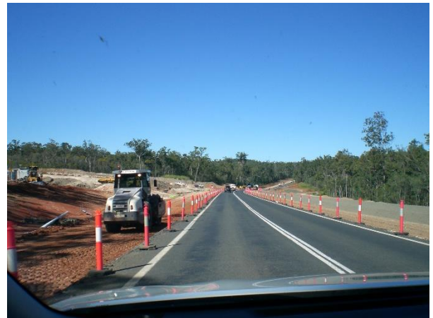
Roadworks south of Gin Gin
