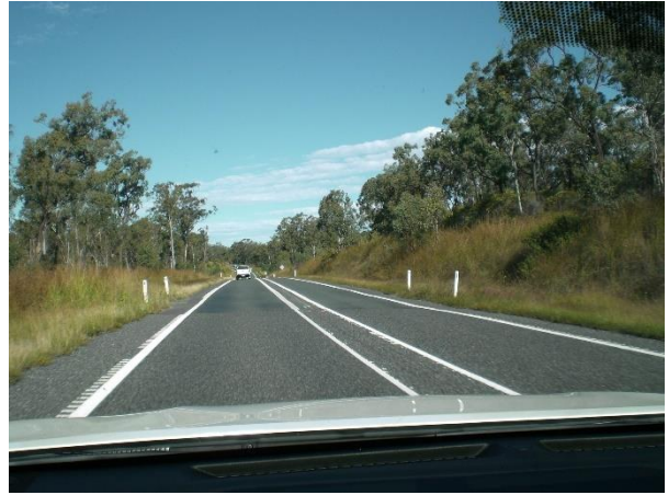
Deteriorated ALTM
