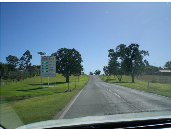
Example of Connected Infrastructure
