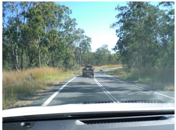
Narrow lane and shoulder
