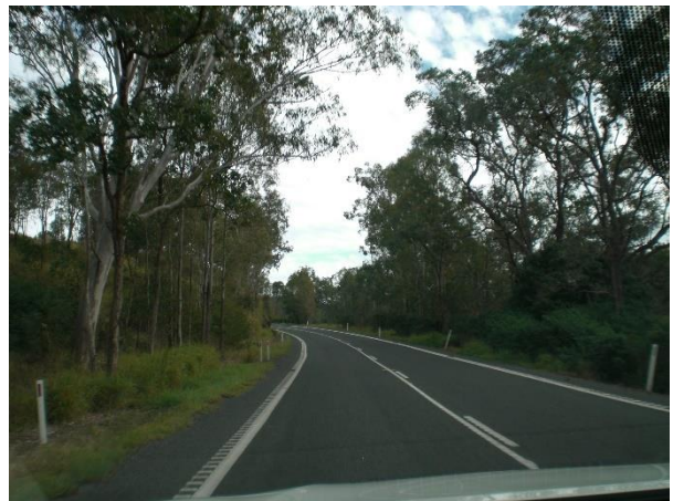
Narrow and roadside hazards present
