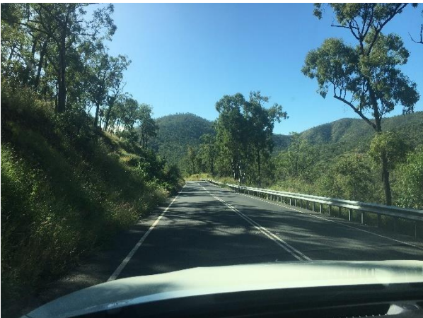
Narrow lane, narrow shoulders and steep embankments
