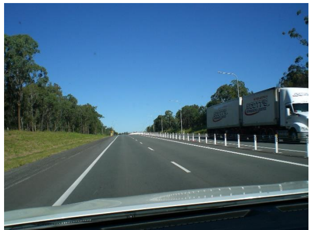
Wire barrier in centreline and wide shoulders
