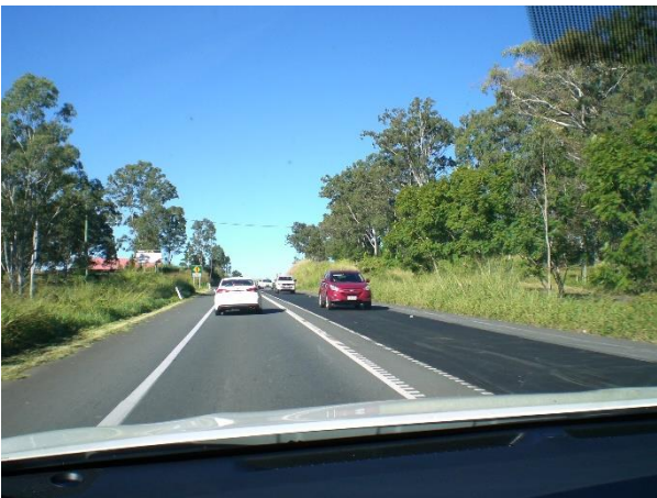
Evidence of road maintenance, north of Gympie
